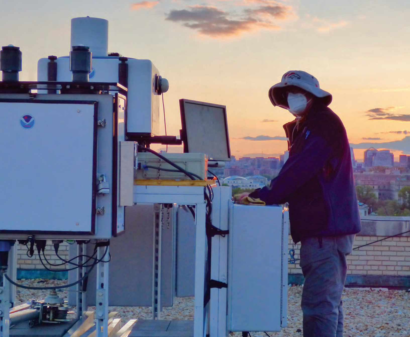
Scott Sandberg, an electrical engineer with NOAA's Chemical Sciences Laboratory, worked with Tyler Boyle of NIST to install a Doppler lidar instrument on April 16, 2021, on top of the Department of Commerce's Herbert Clark Hoover Building in Washington, D.C. for a research project studying urban greenhouse gas emissions. Credit NOAA's Scott Sandberg and NIST's Tyler Boyle
